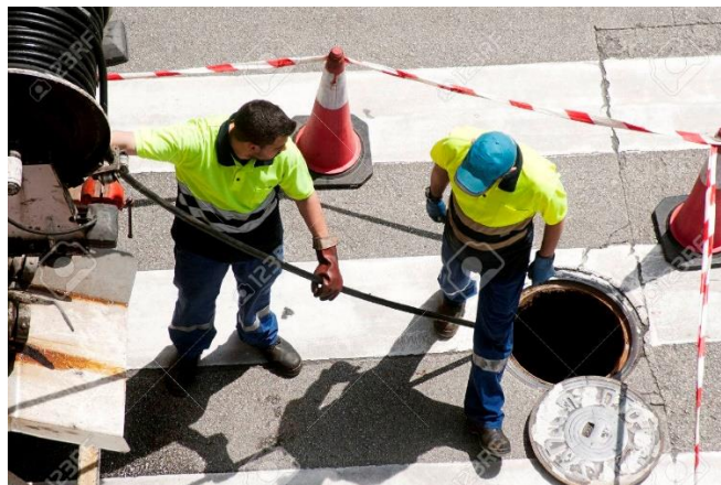
Hydrogen sulfide gas can be created in sewers when bacteria break down human waste. If a sewer is uncovered, you may smell a bad odor. (Image source: 123RF Stock Photos)
